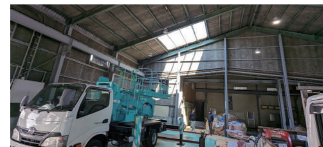
▲倉庫屋根開口工事
